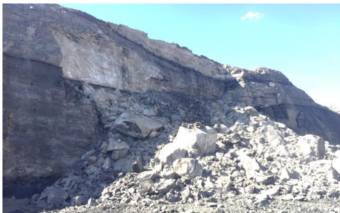
Figure 1 Case study 1, post failure slope conditions
