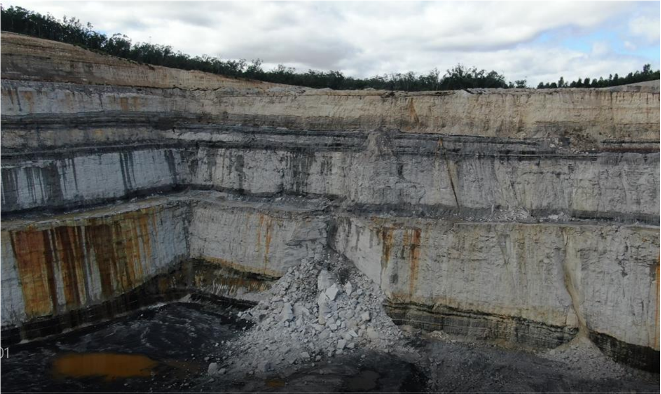
FIG 3 – Highwall Rockmass Failure
